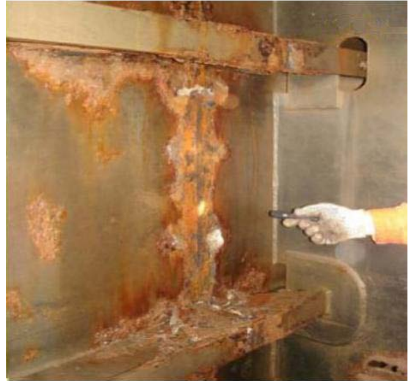
Power-tooled block joint after 5 years service
