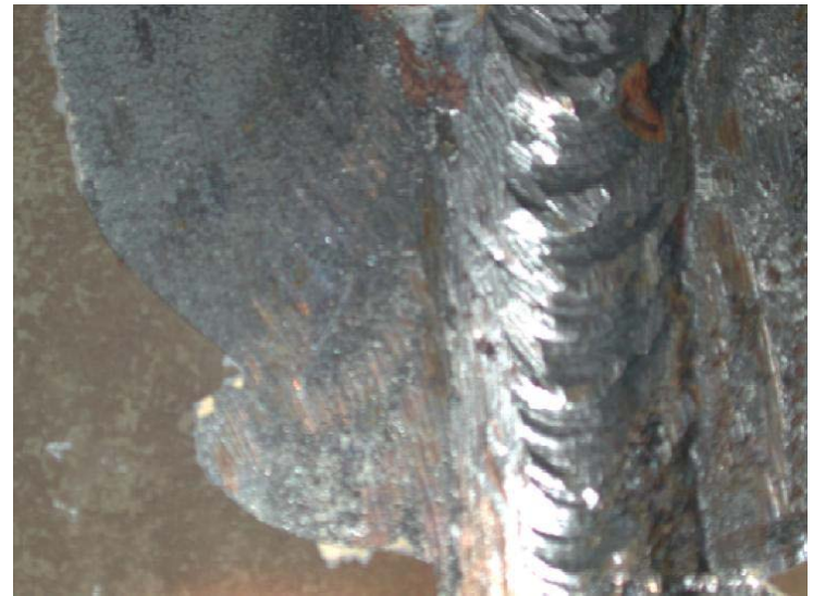
St3 power-tooled surface finish
